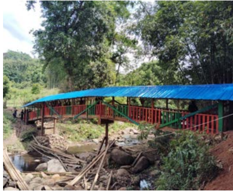
Bridge constructed in Yeh Mu Plaw area
