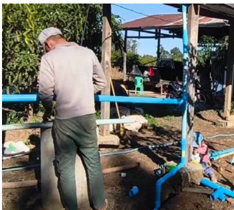
Repairing water pipelines in an earthquake-affected village
