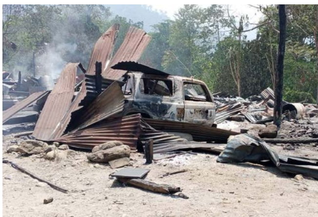
Civilian infrastructure damaged by SAC air strikes
