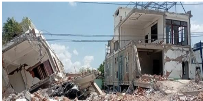
Houses destroyed by earthquake
