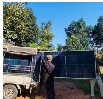
Community members transporting solar panels for installation to the earthquake-affected communities.
