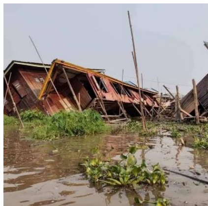
Collapsed houses in the Inle region following the March 2025 earthquake
