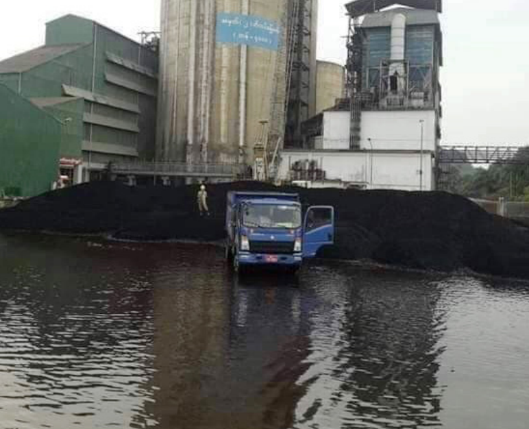
Photo taken early in the 2019 flood season showing one of the 2 coal piles in the 4000 TPD cement plant soaking in water that has turned totally black.
