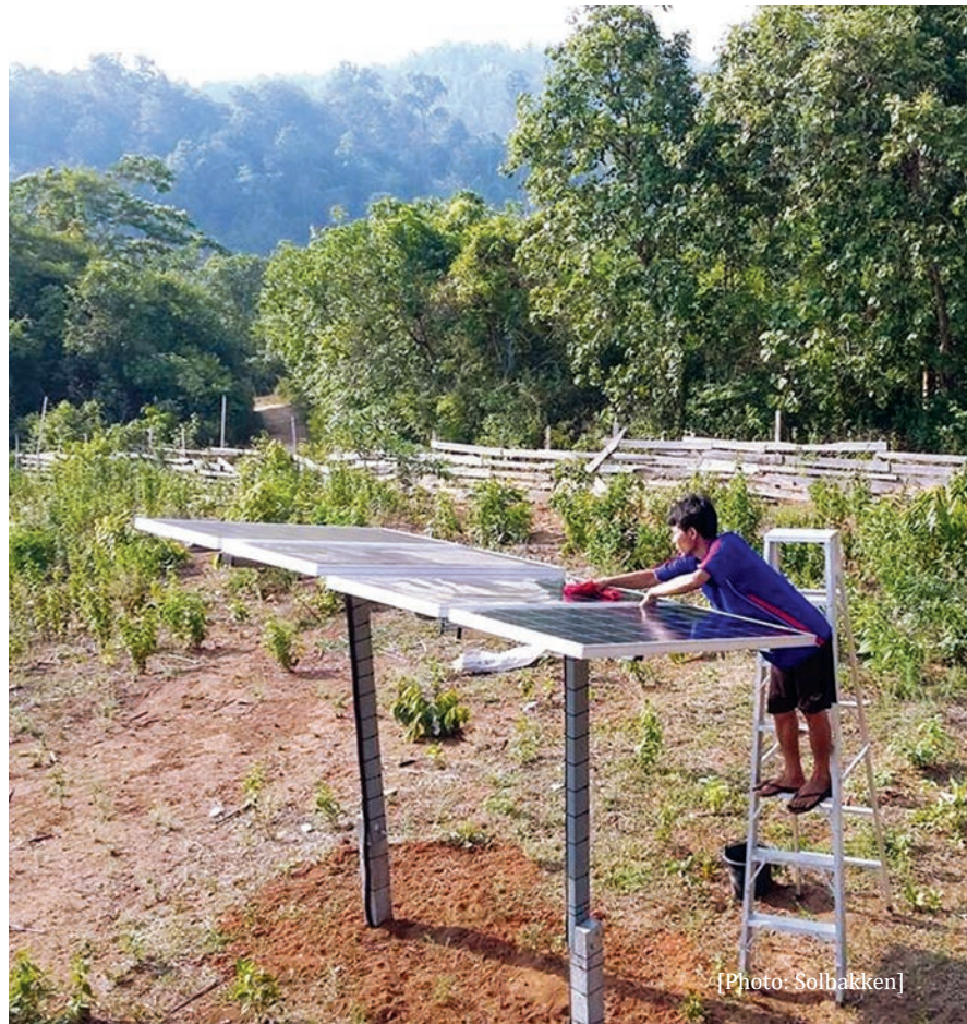
Maintenance of solar panels in Karen State.
