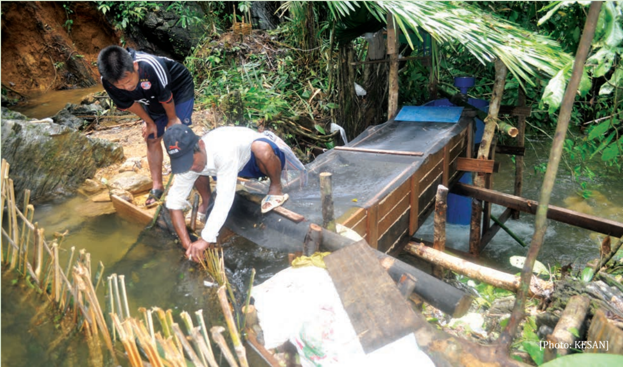
Community members in Kwelapya Village in Beelay Township, Doo Tha Htoo District in Karen State are building a micro-hydro power system.
