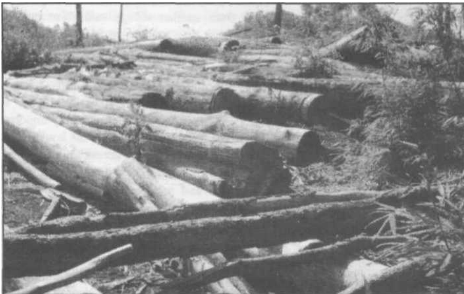
Clear-cut for future dam development
